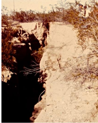
Earth Fissure in Chandler Heights in 1978, it is some years old and eroding. Unfortunately, people used the fissure as a trash disposal site (Chandler Heights).
