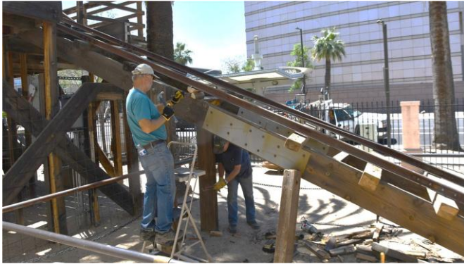
Bill L. and Don remove old ties from the incline.
