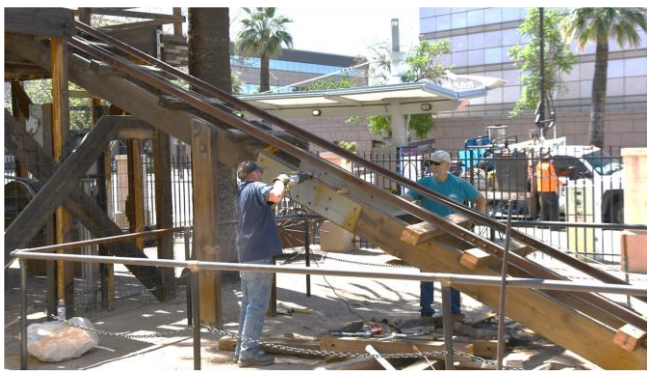
Bill L. had to cut the old lag bolts.
