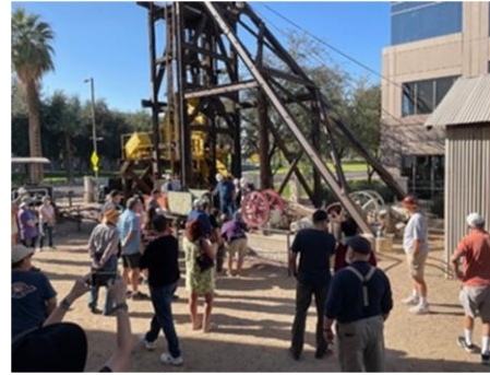
Boras Headframe The Boras Headframe was the last of the wooden headframes built in the Warren Mining District near Bisbee, Arizona. Erected in 1917, it hoisted over 50,000 tons of copper ores by 1926 when the mine was closed during the Depression. Production resumed in 1938 and continued to 1941. In 1952 the headframe was reconditioned and some of its wood supports were replaced with steel. Until 1975 it served as a ventilation and escape shaft for the interconnecting underground workings of the Dallas and Cole mines. The relocation to Phoenix was completed in 1997.
