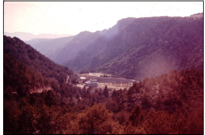
The top of the travertine dam filling in Pine Creek Canyon, the bridge is under this flat surface.
