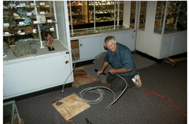
Jerry adding electrical wiring for the cases in the main gallery
