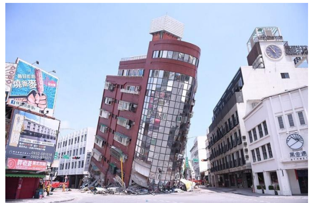
Earthquake Damage in Hualien City, Taiwan
