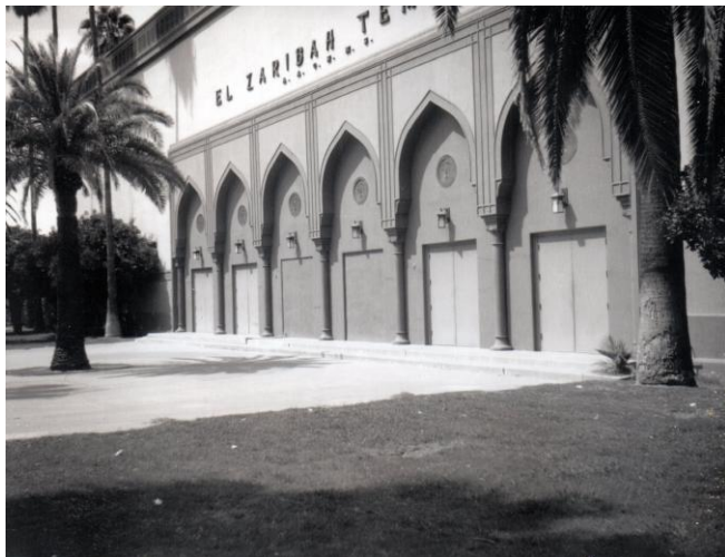
A pre-renovation photo of the south side of the 'El Zaribah Temple' facing Washington St.
